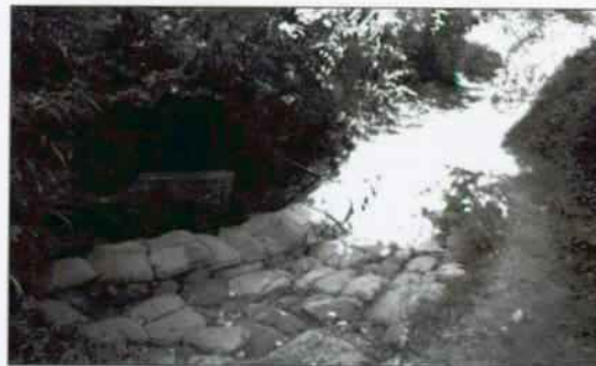
Figure 94 In the summer of 1997, eroded path and the stream bank were stabilized by the Student Conservation Association, August 1997. NCR, Photo Archive, DOP 42-14a.
