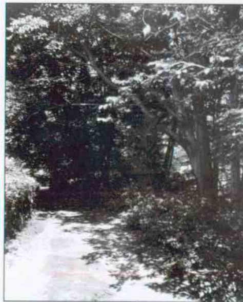
Figure 83 Beech Grove corridor as it appeared in the summer of 1932. DOSLA, Photo Archive, #13.27.
