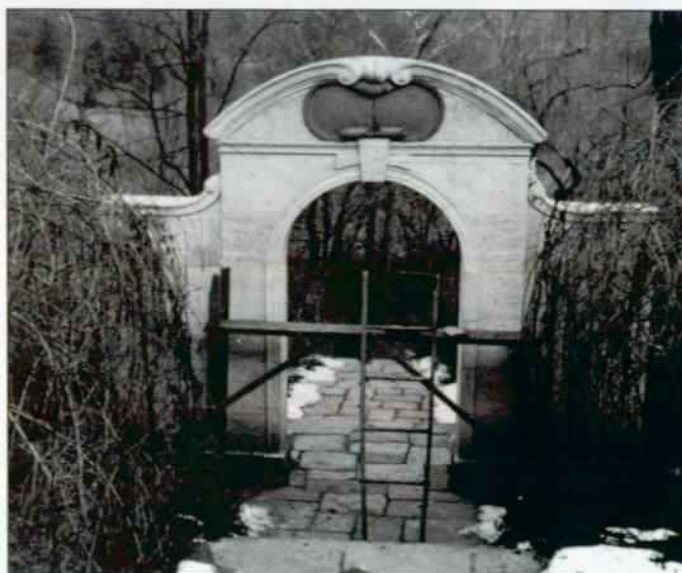
Figure 21 Construction of Forsythia Arch, ca. 1938. DOSLA, Photo Archive, #17.13.
