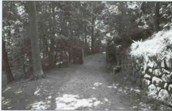
Figure 158 View of the Beech Grove retaining wall and Lovers' Lane gate, August 1997. NCR, Photo Archive, DOP 40-2.
