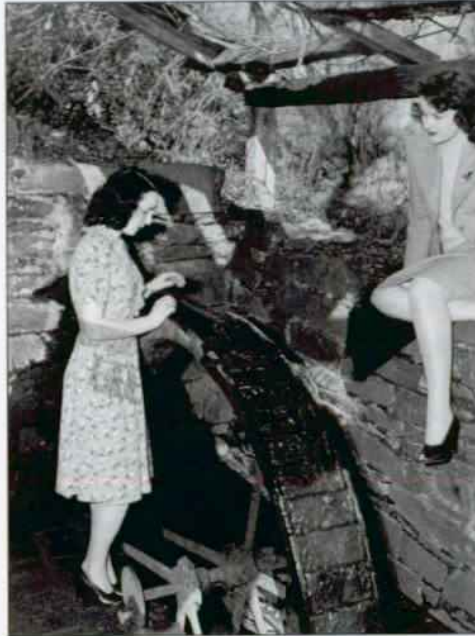
Figure 166 Deteriorated Old Pump House with water wheel broken into pieces as documented by the NPS, 1976. NCR, List of Classified Structures (LCS), Photo Archive, Rock Creek Park.
