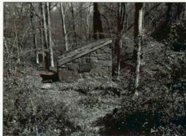
Figure 162 View of west side of Old Stone Pump House, April 1, 1997. NCR, Photo Archive, DOP 2-35a.
